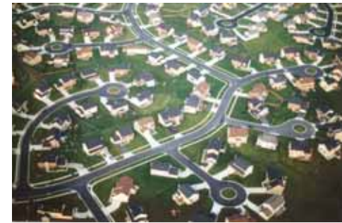
New residential development without a focal point, green network or variety of scale in streets and homes.
