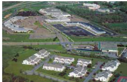
Village scale mixed-use area with no core, no focal points or open space. Car is king.
