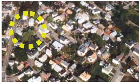
Civic focal point anchoring dynamic neighborhood - hierarchy in land use and street types.
