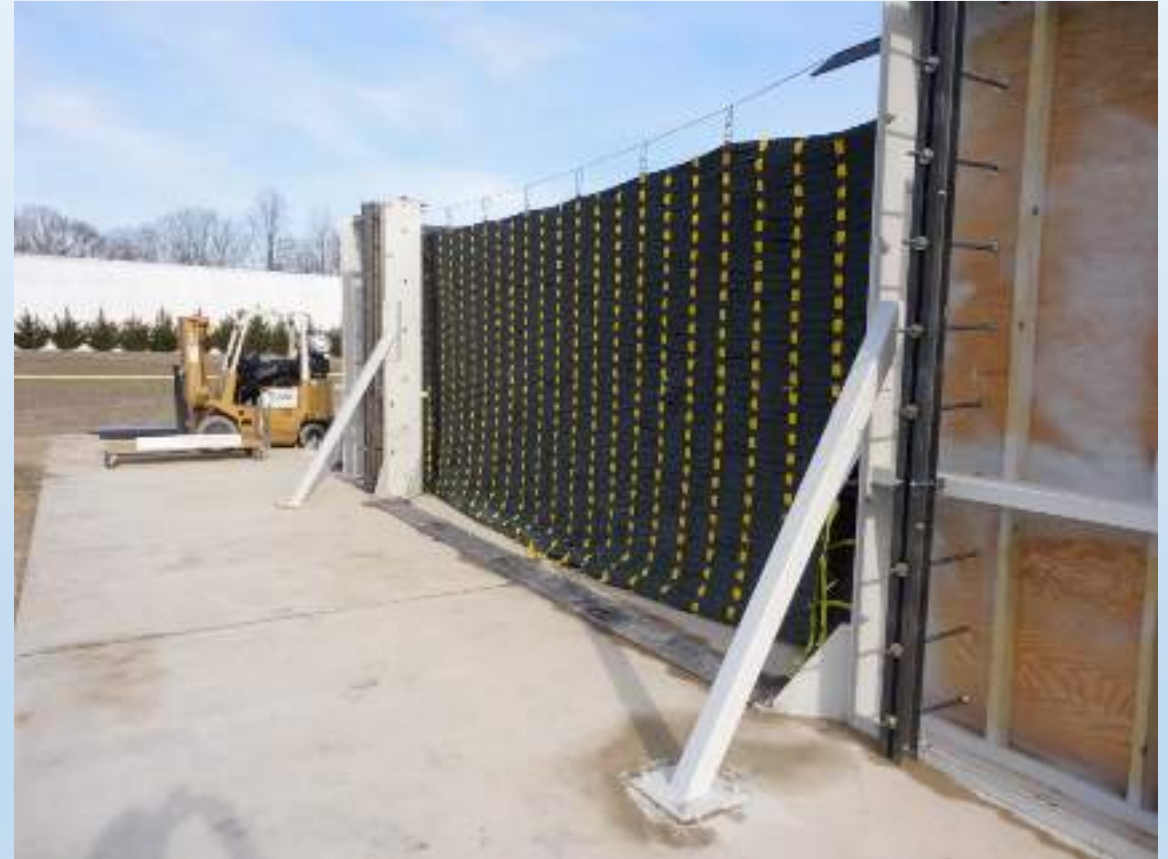
ENTRANCE CLOSURE OR BUILDING ENCLOSURE ILC DOVER – FLEX WALL
