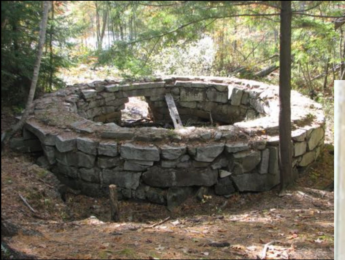
Foundation of a Powder Mill at Gambo
