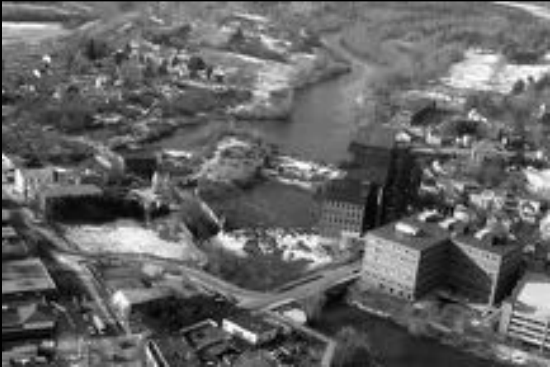
Saccarappa Dam Complex, Westbrook
